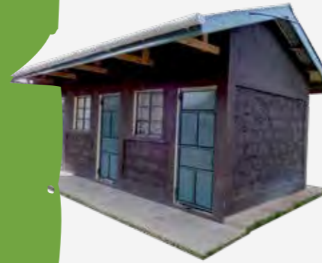
new accommodation blocks, each with three housing units, built for our wildlife rangers
