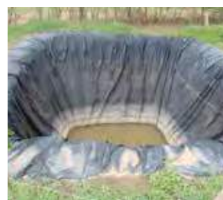
water pan constructions
